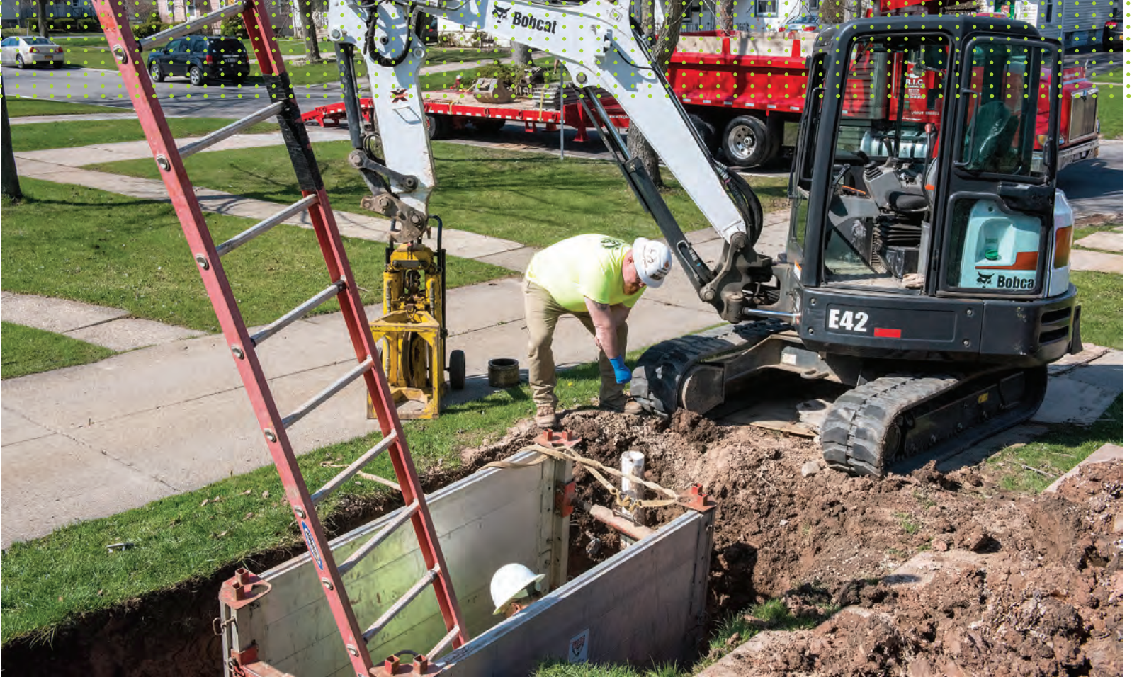
↗ Company co-owner Adam Kuhns checks the trench after placing a shoring device.
