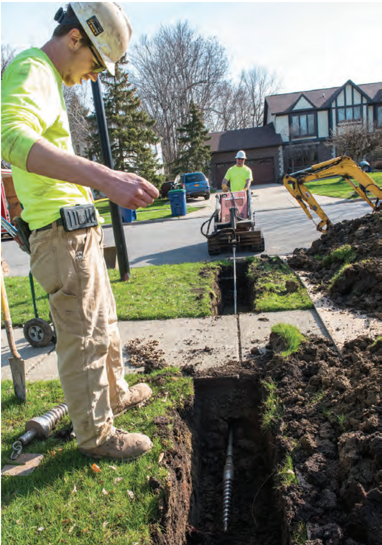
↗ Company co-owner Adam Kuhns checks the trench after placing a shoring device.
